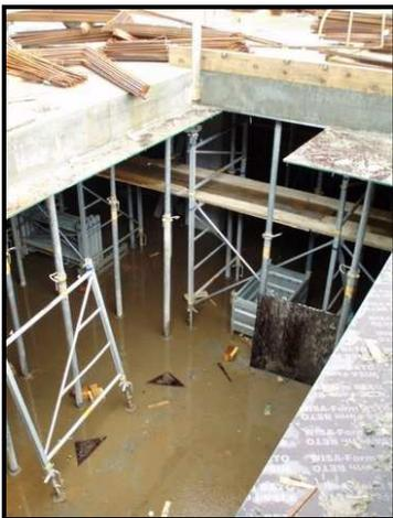
*A construction site worker fell over 13 feet when he climbed under a guard rail onto unsupported formwork*
